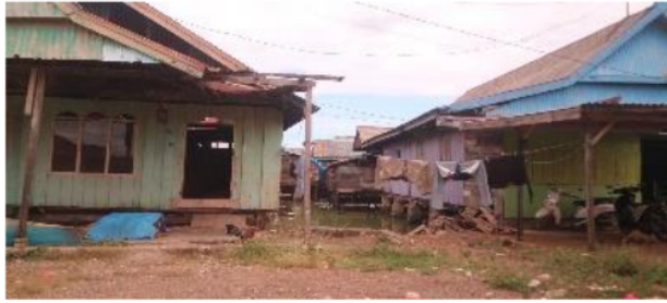
Picture. 9. Condition Sanity in Settlement Patterns Elongated (Linear)
